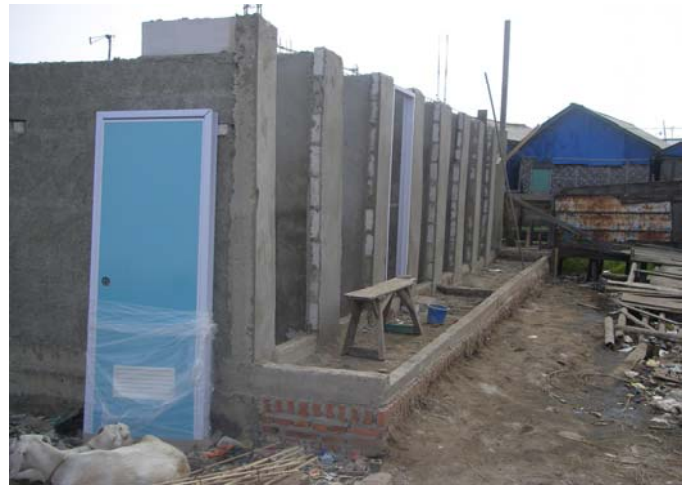
The Public Toilet (After)
