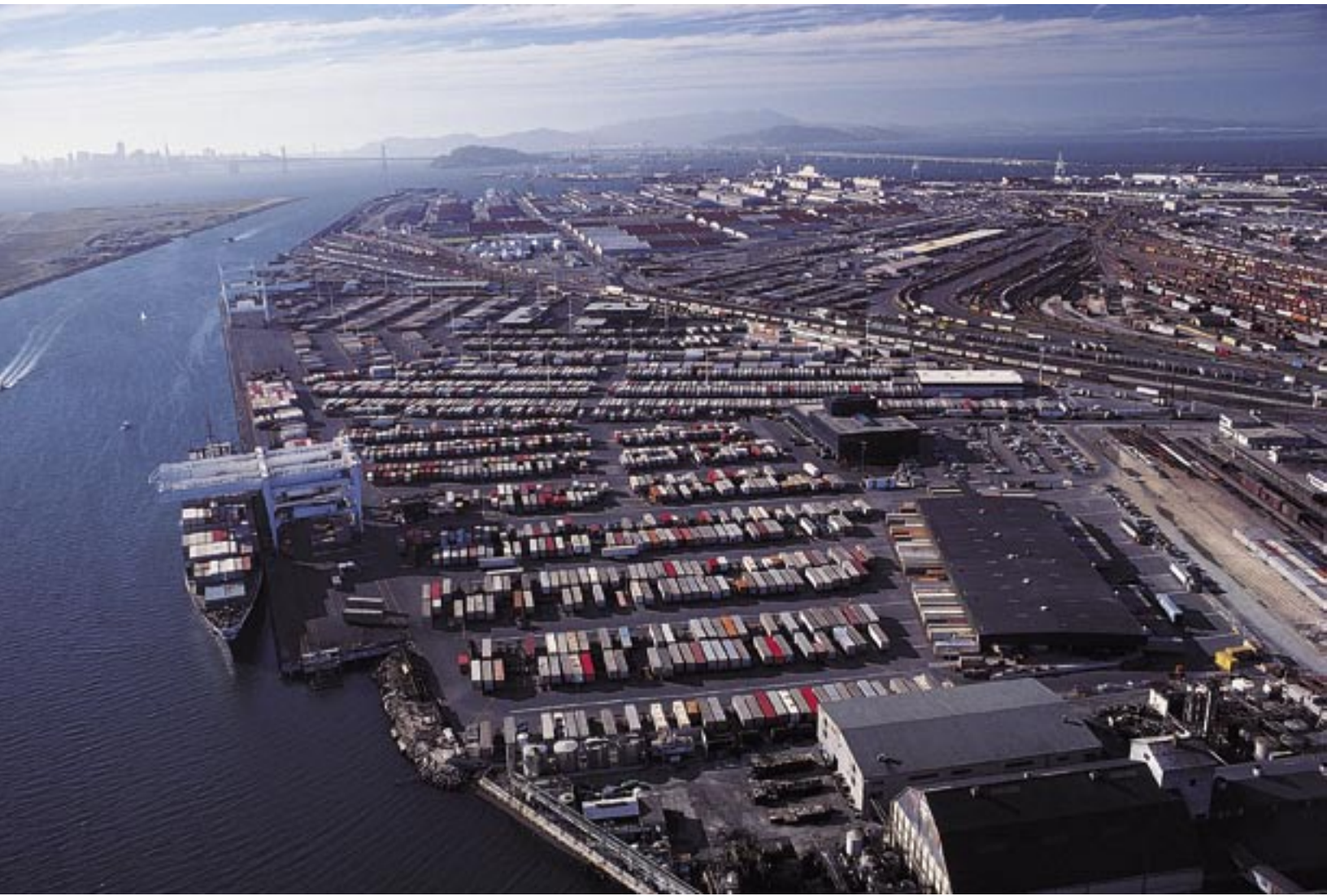
Port of Oakland, California
